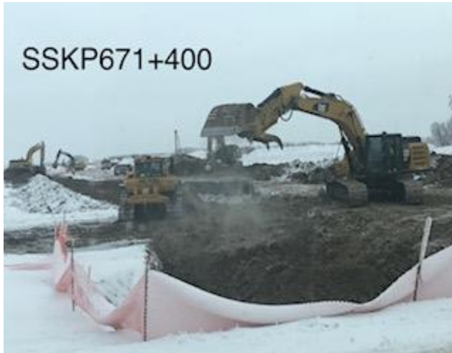
Bell hole backfill and wet land compaction
