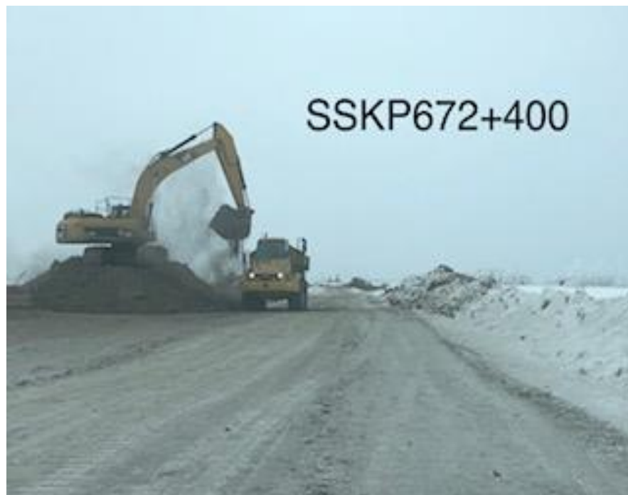
Backfill at Water Course Crossing SK WC74
