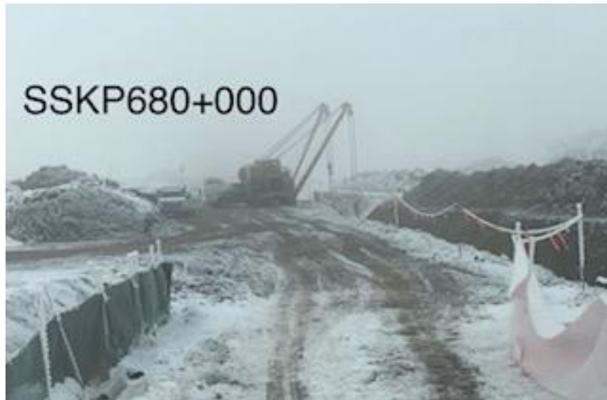
Lowered in a joint section and tie in – organic field
